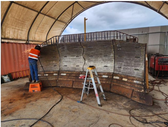
Field repair of a dozer liner package with QARC™ wire
